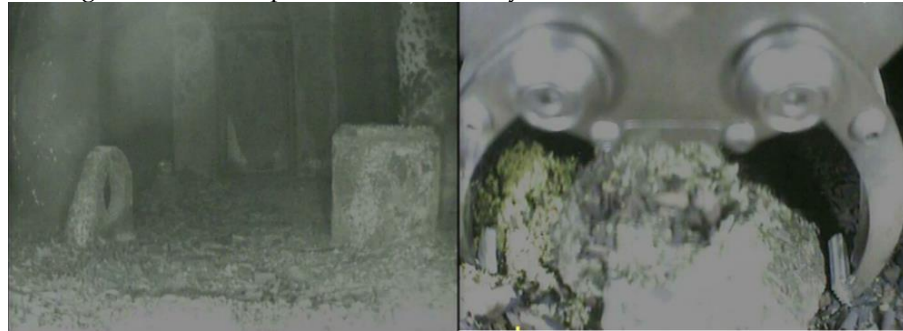
Figure 2. Photo from the hot gas chamber of the KS 150 reactor.
