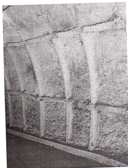
*Figure 3 Image of the combined substructure of steel frame and sprayed concrete
