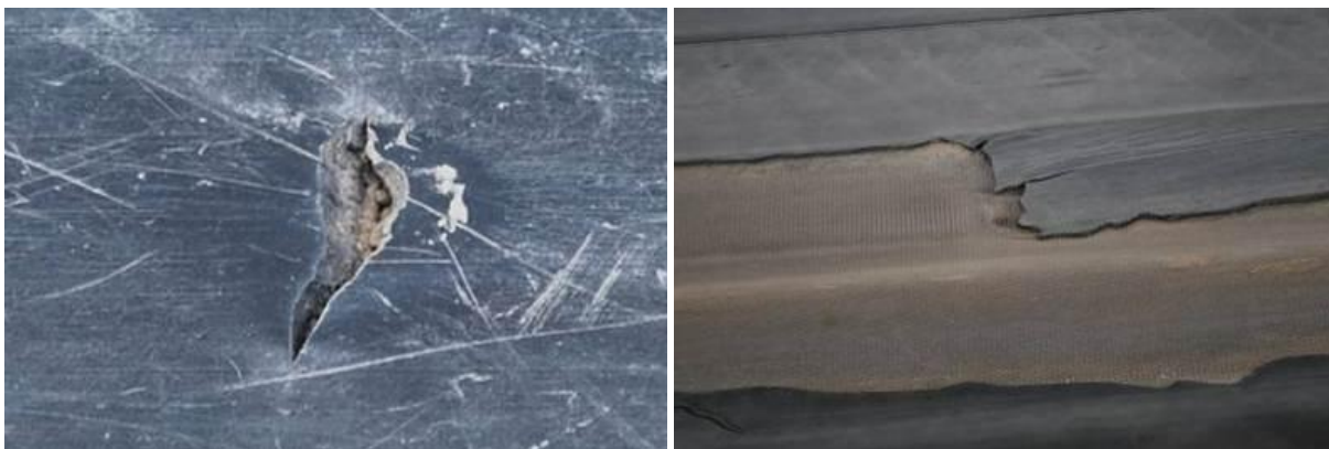
Figure 1 Damages of the conveyor belts – SD a.s. Bilina surface mine
