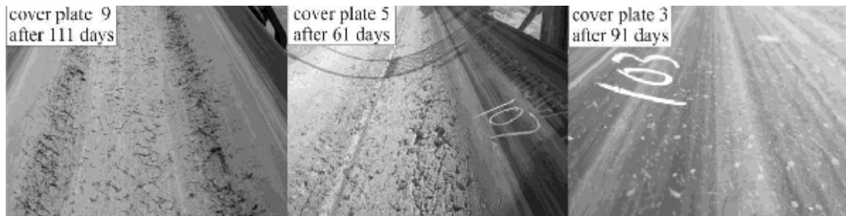
Fig. 3 Cover plate damages in field tests
